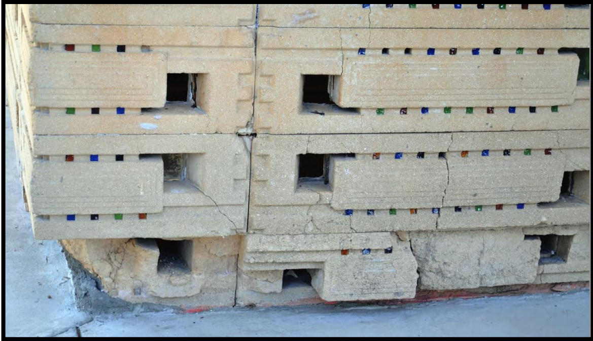
Fig. 32 Cracking, erosion and deterioration are unmistakable in this view of the corner of blocks. Surface water appears to be the leading cause of damage to the ground level. Jeffrey M. Chusid, World Monument Fund.
