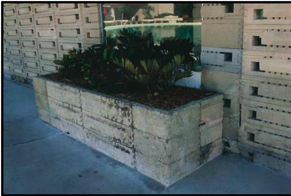
Fig. 13 Damage to the Three Seminars is inclusive to widespread discoloration, deterioration and biological staining from moisture damage. Mesick Cohen Wilson Baker Architects
