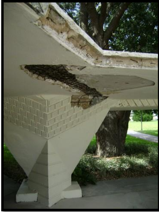
Fig. 27 Cracking, deterioration and sagging, as viewed in the esplanades, are caused by rusted and corroded steel reinforcement and the lack of design of expansion joints. Mesick Cohen Wilson Baker Architects.
