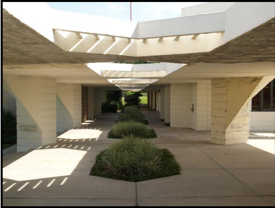
Fig. 26 View of an esplanade. The entire system of walkways was completed in the 1950s. There is evidence of biological staining on the ceiling, stripping of the paint and cracking due to lack of expansion joints. Cambridge 2000 Gallery , http://www.cambridge2000.com/gallery/html/P72021532e.html .
