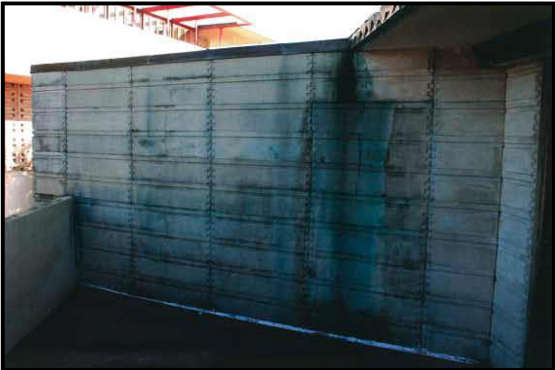
Fig. 25 William H. Danforth Chapel, east façade is host to biological staining, copper carbonate deposits, and improper repairs with sealant. Mesick Cohen Wilson Baker Architects.
