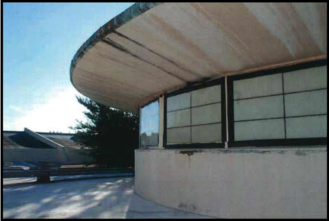
Fig. 20 Fletcher Theater housed in the Industrial Arts Building, damage includes corrosion of metal elements and concrete deterioration. Mesick Cohen Wilson Baker Architects.
