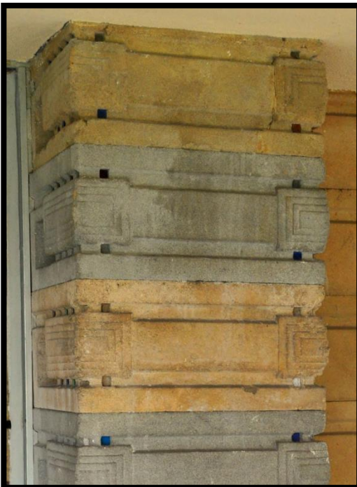
Fig. 30 Another example of discoloration due to different mixes and replacements of blocks. Also there are hints of biological staining and efflorescence. Jeffrey M. Chusid, World Monument Fund.
