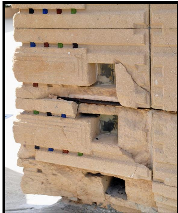
Fig. 31 Thermal expansion of the corner blocks has been a primary cause for the apparent cracking. The steel reinforcement is rusting and corroding, as well, causing the blocks to further deteriorate. Jeffrey M. Chusid, World Monument Fund.
