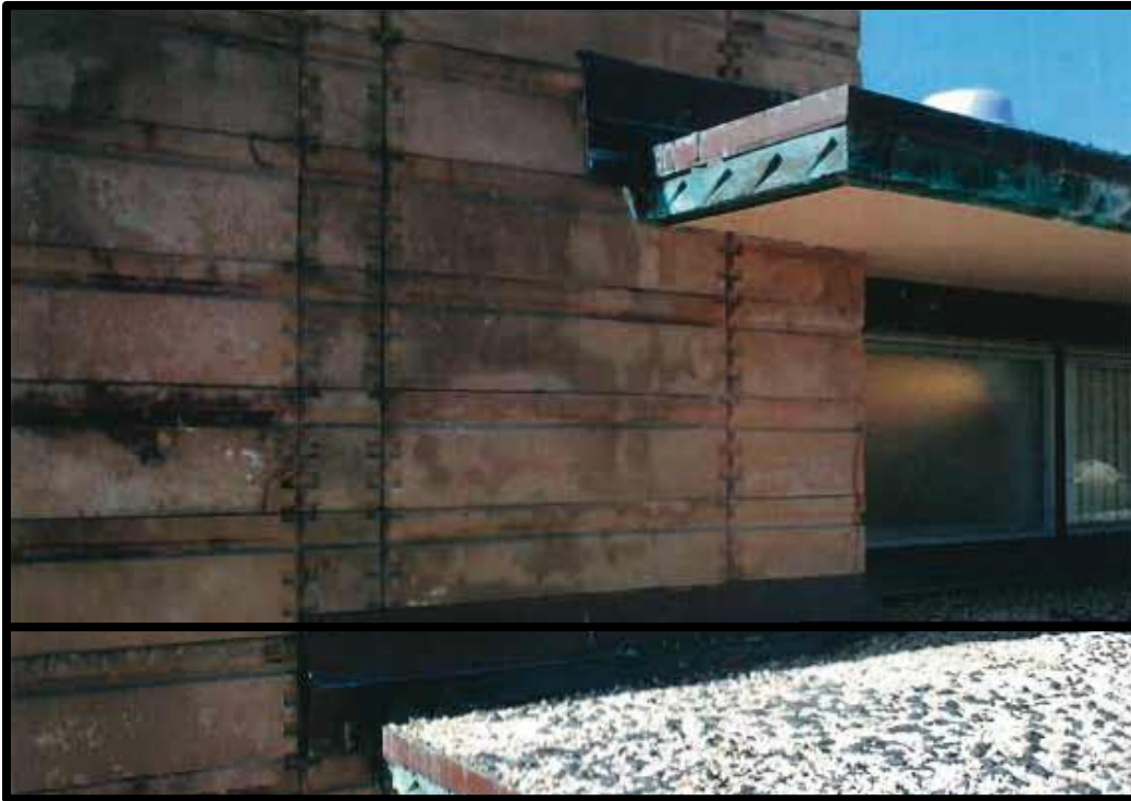
Fig. 22 Polk County Science Building, east façade shows biological staining and mold from moisture infiltration. Mesick Cohen Wilson Baker Architects.
