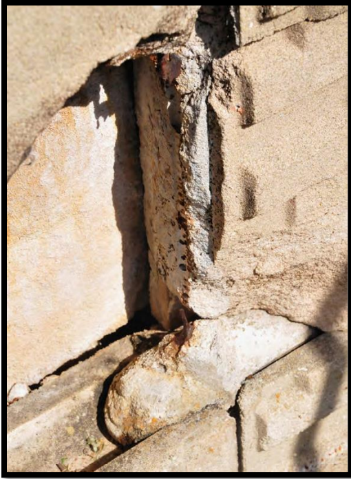
Fig. 28 The steel reinforcement has caused erosion, instigating the brick to lose its integrity, now highlighting the once hidden grout tubes. Jeffrey M. Chusid, World Monument Fund.
