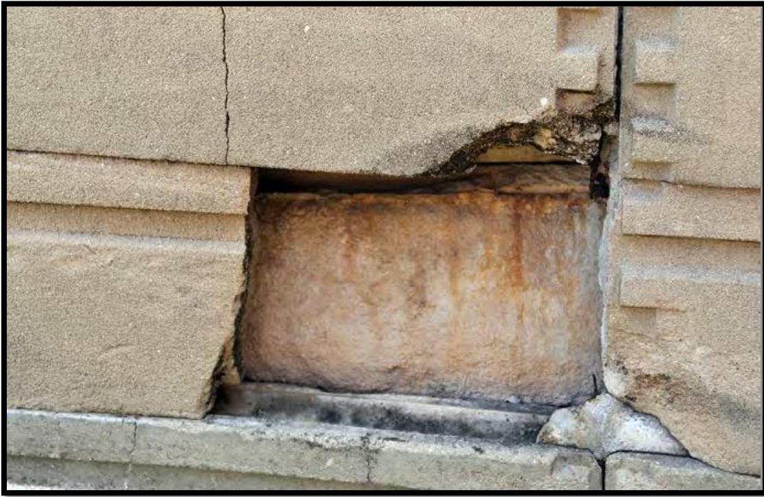
Fig. 33 Example of the facing separating from the block system. Jeffrey M. Chusid, World Monument Fund.
