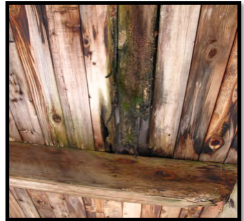
Fig. 2.21 Water damage on the rafters and eaves.
