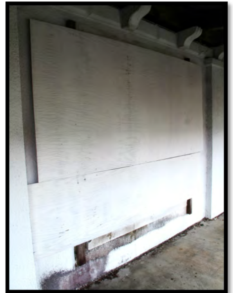
Fig. 2.20 Mildew from water damage under one of the boarded windows on the second-floor of the south façade.
