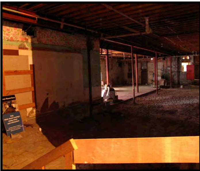
Fig. 2.22 Main Street Leasing's makeshift office space is to the left. Walls are heavily damaged and a rectangular portion of the floor is missing. The ceiling is unfinished.
