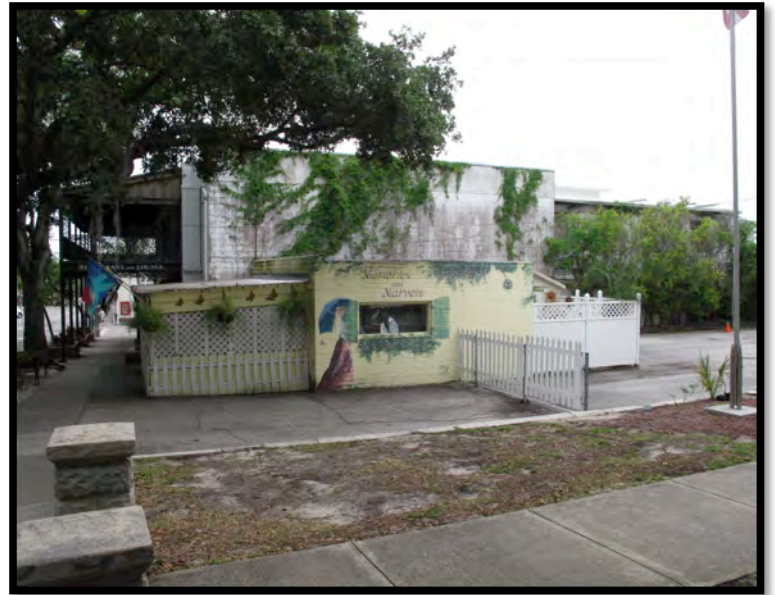
Fig. 2.3 Mildew and overgrowth of vegetation have taken over most of the north façade.
