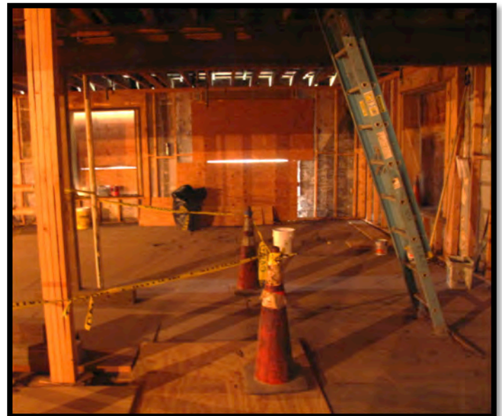
Fig. 2.29 Southwest corner on the second-floor. The wood subfloor is covered with plywood where flooring is missing. The roof is accessible from the ladder
