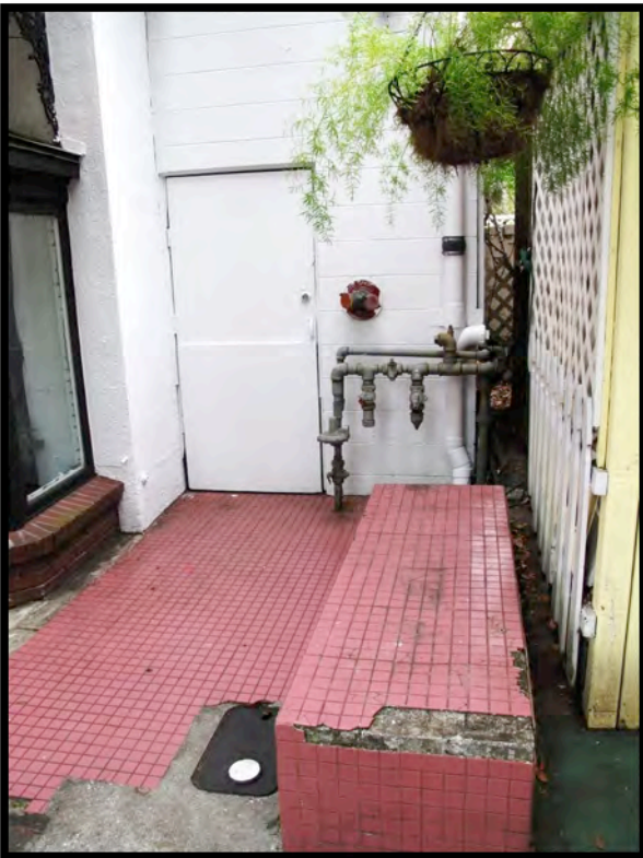
Fig. 2.12 Access door on the ground floor of the northeast corner of the Donnelly Street façade. Exterior tiling has been worn down.
