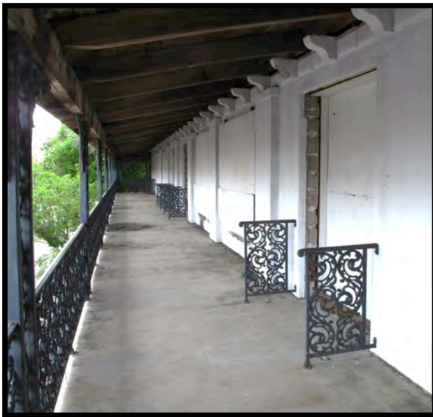
Fig. 2.15 Windows and doors on the second floor of the south façade. Concrete blocks are exposed to the exterior.
