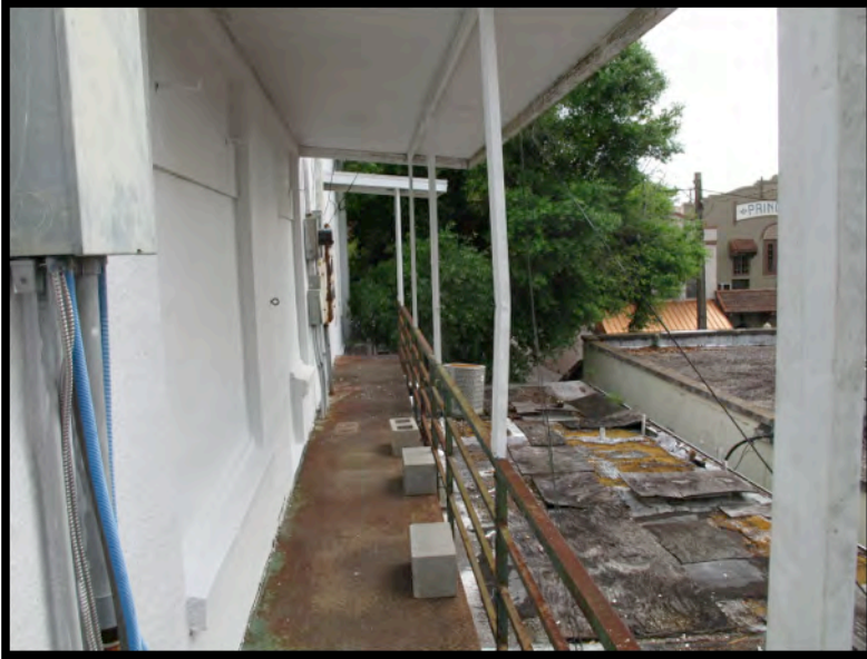
Fig. 2.8 Rusted iron balcony on the west façade. The roof of the rear bathrooms, to the right, is situated in a connected outbuilding
