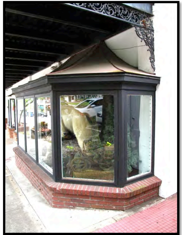
Fig. 2.17 One of the projected bay windows, this one is projected 4' east of the building towards Donnelly Street. A metal roof covers the extended bay window and an aluminum-cast framework sits atop a brick foundation.
