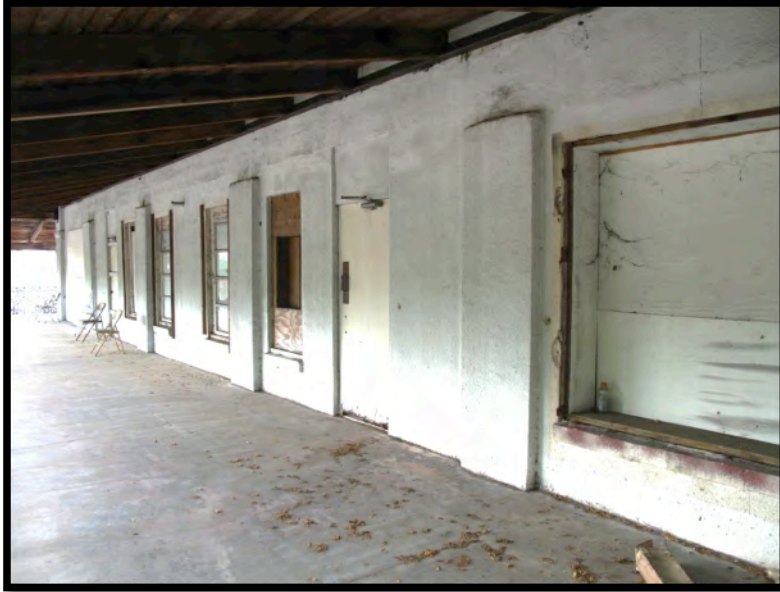
Fig. 2.13 Windows and doors on the second-floor of the east façade, facing Donnelly Street. The door to the to the far left is blocked from opening. There are four windows and/or frames in the middle and another 4' x 6' window to the far left.
