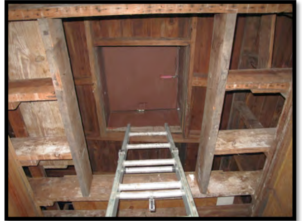
Fig. 34 The roof is accessed through this opening and the use of a ladder. The water damage is evident in the joists above.
