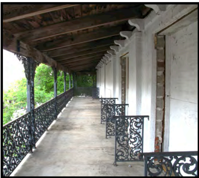
Fig. 2.6 Second-floor balcony on Fifth Avenue looking west. The stucco around the doorway has been damaged from water damage. Rafters and eaves above are also damaged from excess moisture.
